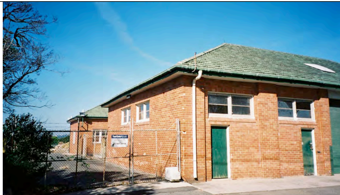
Current view of east façade of Building 7, with Building 6 in the background (Photo: Robertson & Hindmarsh Pty Ltd, 2006)
