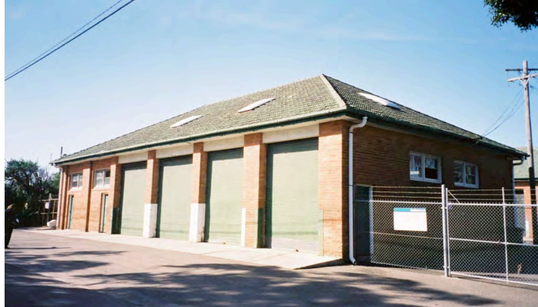
Current view of north façade of Building 7 (Photo: Robertson & Hindmarsh Pty Ltd, 2006)
